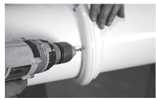
**10.** With the rings properly positioned on the 8" straight post, drive #8x2" self-drilling screws into the post through the holes in the top of the ring, as shown. Slide the top and bottom trim over the post, followed by the top and bottom mounting brackets.
