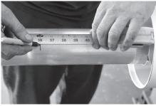
7. Before pre-assembling column, you must determine the placement of the spacers. Measure from the bottom of the aluminum insert (34" for 36" high railing and 40" for 42" high railing). This will be the placement of the bottom of the aluminum insert spacer.
