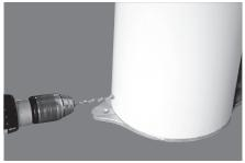
12. In areas where uplift from high winds is considered a problem, pre-drill 1/4" holes through the column and bracket ears at the position of the bracket mounting tabs into the post approximately 1" from the bottom and 1" from the top.
